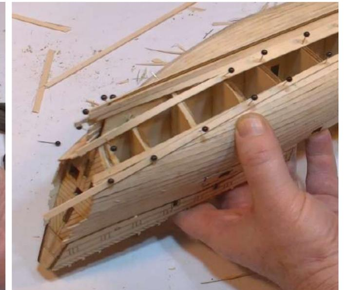
**Step 11** You will reach a point where the remaining gap at the mid-ship area is approximately 8mm - 2 plank width. The gap across the fore planks will be less than 8mm while at the stern the gap will be greater than 8mm. Across the fore gap measure 8mm for the temporary 3rd plank from the keel and mark this width at each fore bulkhead on the last plank fitted.
