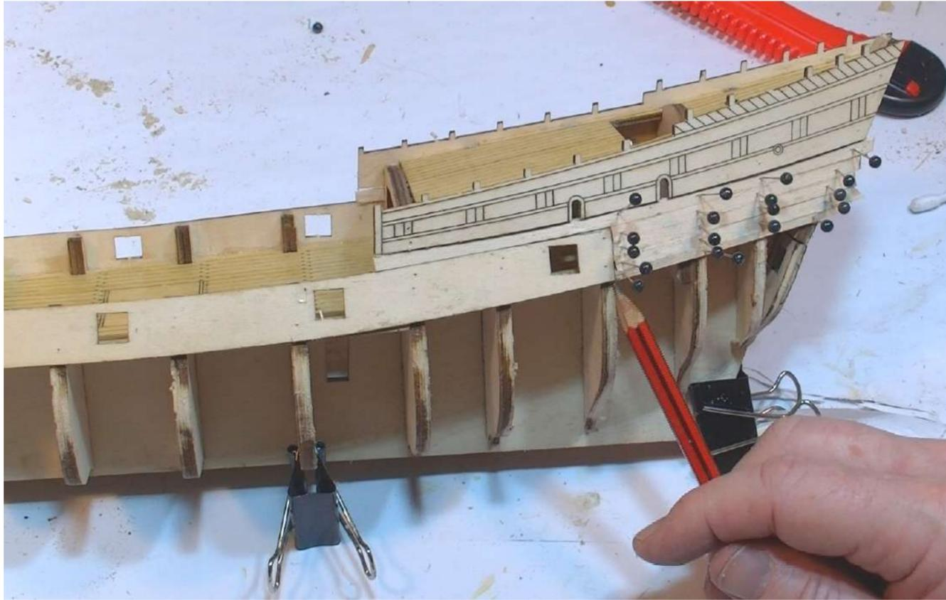
**Step 2** Trial fit a length 1x4mm limewood P24 along the full length of the hull immediately below the bulwark and aft planks as shown - this will be the first plank. Do not taper this plank. Use a plank bender to bend the plank to fit around the bow - start bending from about bulkhead 1. Once satisfied with the fit glue and pin the plank in place. Repeat for the other side of the hull. Make sure the two planks fitted are symmetrical at the bow.
